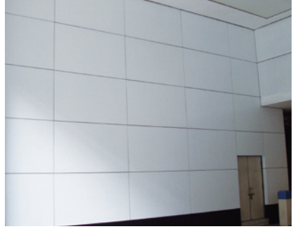
Panel fixed by metal dowels and fixings onto a wall inside a building
