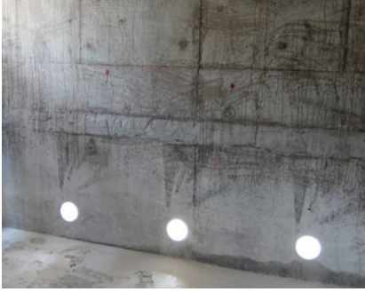
Formation of wall opening
