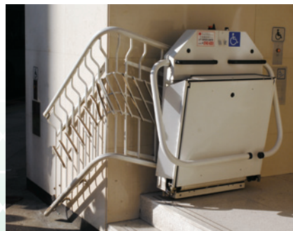
Building works associated with stairlift or lifting platform
