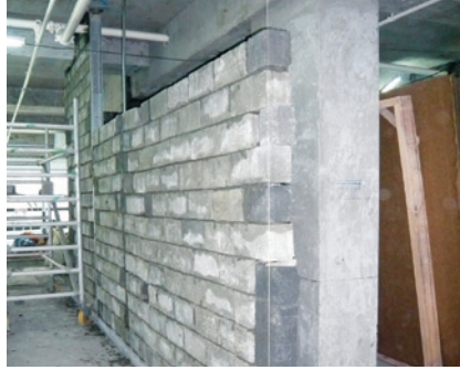
Non-load bearing block wall
