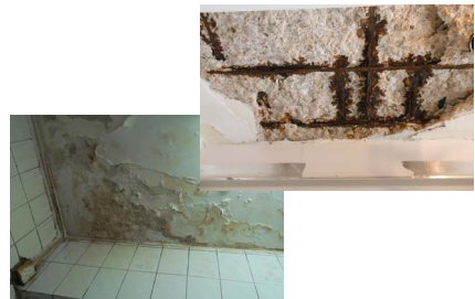
Inadequate or damaged waterproofing may result in water seepage and spalling of structural elements
