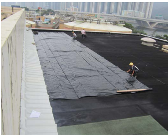
Proper installation, protection and upkeep of waterproofing layer on roof/podium
