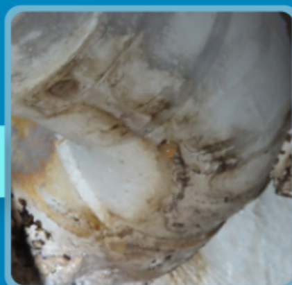
外牆排水管滲漏或破爛 Leaking or broken drainage pipes at external wall
