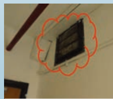
於逃生樓梯或其防護門廊 牆身開鑿開口 Formation of openings to the walls of the escape staircase or its protected lobby
