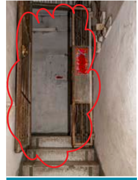
加裝捲閘，或安裝不適當 的鐵閘或被上鎖，導致阻礙 逃生通道 Obstruction to escape routes caused by addition of shutters, inappropriate installation of metal gates or locked metal gates
