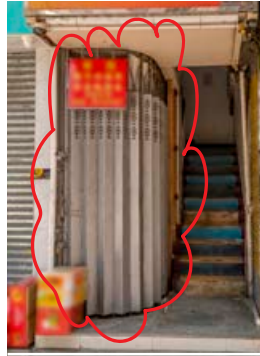
於逃生樓梯或其防護門廊內加建 僭建物，例如梯底舖 Addition of UBWs at the escape staircase or its protected lobby such as under-staircase shops
