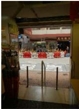
於逃生通道安裝固定裝置 導致出口闊度不足 Inadequate width of exits caused by installation of permanent features on escape routes
