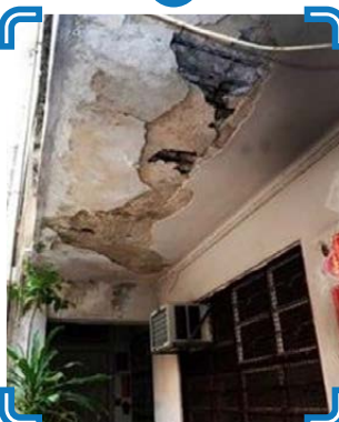
鋼筋外露生鏽 Rusting of Exposed Steel Reinforcement
