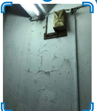
批盪剝落 Detachment of Plastering
