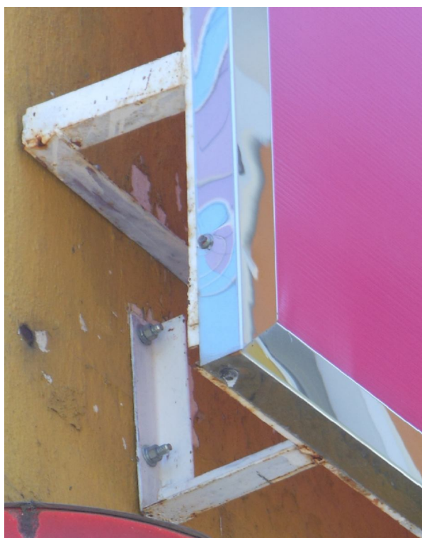
照片3: 招牌的支撐點A7 (支撐點A1, A4及A10皆類同)
