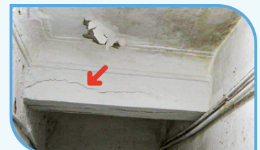
Longitudinal crack along the steel bar in concrete
