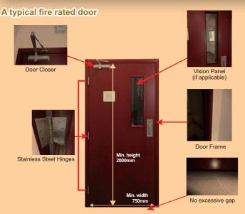
\* The design details of different brands of wooden or glass fire rated doors may vary but they should be constructed in accordance with all requirements, including dimensions, ironmongery works and intumescent strip, as stipulated in the test reports before it can be accepted.
