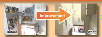
Services inside escape staircases, e.g. electrical cables and meters, should be enclosed by fire rated materials to prevent the spread of fire from such services. No enclosures are required for optical fiber wires, water valves and water meters.
