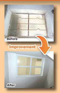
Fixed lights with fire resistance period of not less than half an hour shall be provided to prevent the spread of fire from the windows of adjoining buildings or other windows of the same building.
