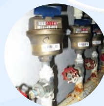
Test for water supply pipes
