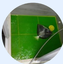
Ponding test for floor slabs
