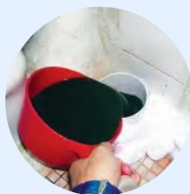
Colour water test for drainage pipes
