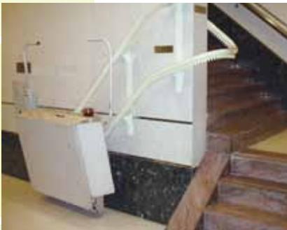
Building works associated with stairlift or lifting platform
