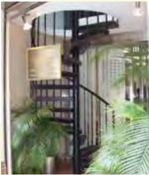
Internal staircase and formation of slab opening
