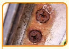
Broken, loose, rusted or missing rivets / screws on the top and underside of the window sash
