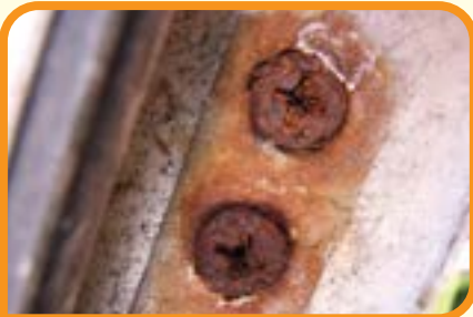
→ Broken, loose, rusted or missing rivets / screws on the top and underside of the window sash
