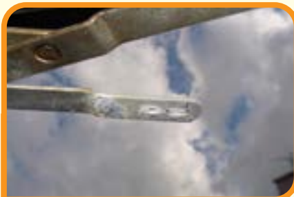
→ Greyish white powder appearing at the hinges, tracks, rivets/screws and locks
