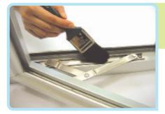
Check regularly and clean the bar hinges and tracks of deposit and sand
