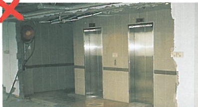
Removal of fireman's lift lobby
