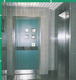
Fireman's lift lobby
