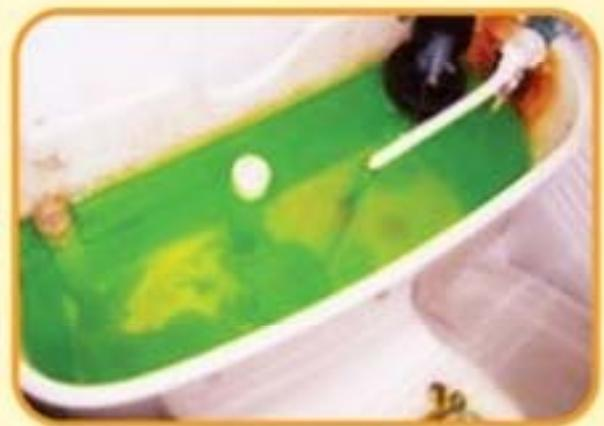
You may apply colour water to detect any leakage in the components of a floor drain, a bath tub or a shower tray step by step (changing the colour to distinguish one test from another) as shown: -
