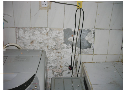
Spalling of tiles
