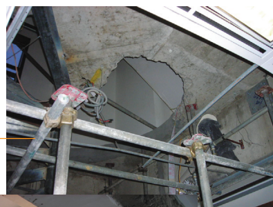
Demolish part of floor slab
