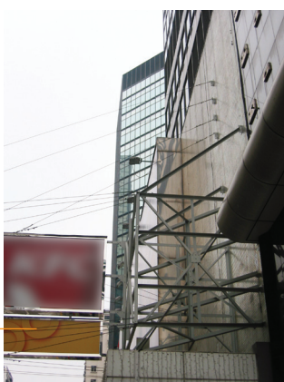
Structural frame of signboard
