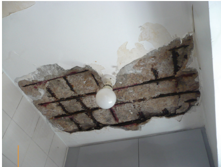
Concrete spalling and rusty reinforcement
