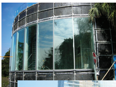
Install curtain wall
