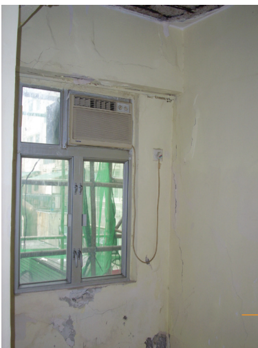
Structural cracks
