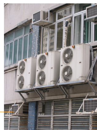
Structural supporting frame for A/C units
