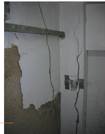
Structural cracks
