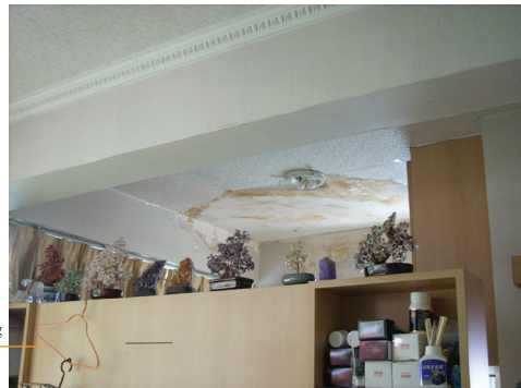
Water stains on ceiling
