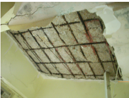
Spalling concrete
