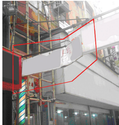
Twisted supporting metal frames
