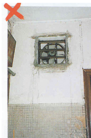
Unauthorised formation of fire resisting wall with installation of exhaust fan
