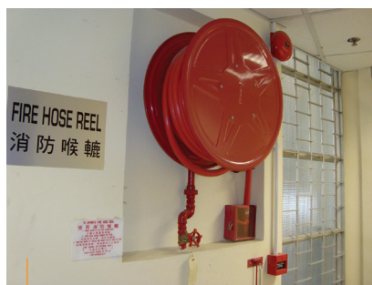
Fire hydrant and hose reel system
