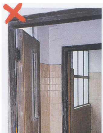
Damaged/Missing fire doors
