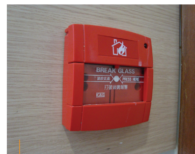
Manual fire alarm system
