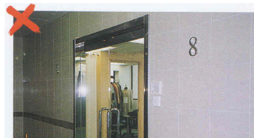
Glass door of inadequate fire resistance open onto the common corridor
