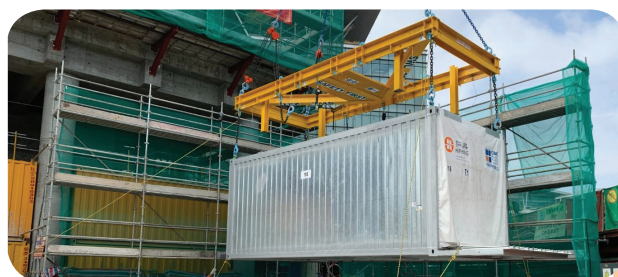
Delivery of MiC module to site
