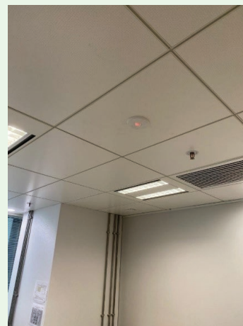
Motion sensor installed in our office
