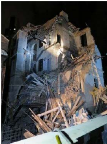
View towards Northwest Elevation
