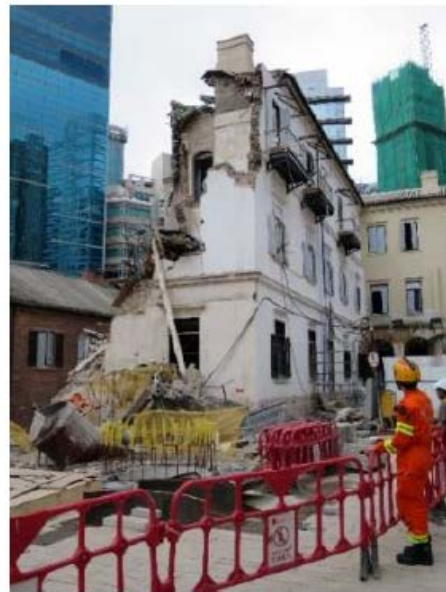
View towards Southwest Elevation
