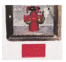
Fire service installations should be kept in good working order at all stages of the works. In case of major works to be carried out to the internal common parts of the building, the existing fire service installations e.g. fire hydrant and hose reel, fire alarm, sprinkler system, etc, should be checked to ensure that they function properly prior to the commencement of the works.
