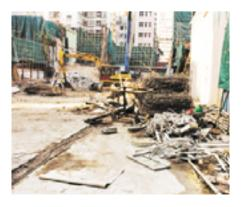
Transportation of materials and debris should be designated and properly specified. Extreme care must be exercised not to allow overloading of any structure or device such as lifts to avoid sudden collapse. In case the use of the passenger lifts is required for the works, the lift car finishes should be properly protected. The use must also be supervised by qualified personnel to avoid overloading.
