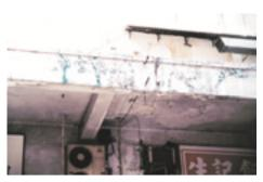
causing serious or fatal injuries if there is lack of maintenance/repair, misuse, addition of UBW above or below the canopies, material corrosion/deterioration, poor construction, etc. There are also cases where the collapsed canopy itself is an unauthorized addition. Overloading the approved balconies by using them for storage leading to eventual collapse have also been found.
