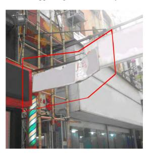
3. Metal supporting frame seriously corroded and display surface tilted.
