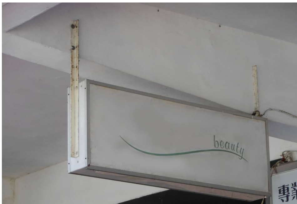
Photo 2: Signboard side view
