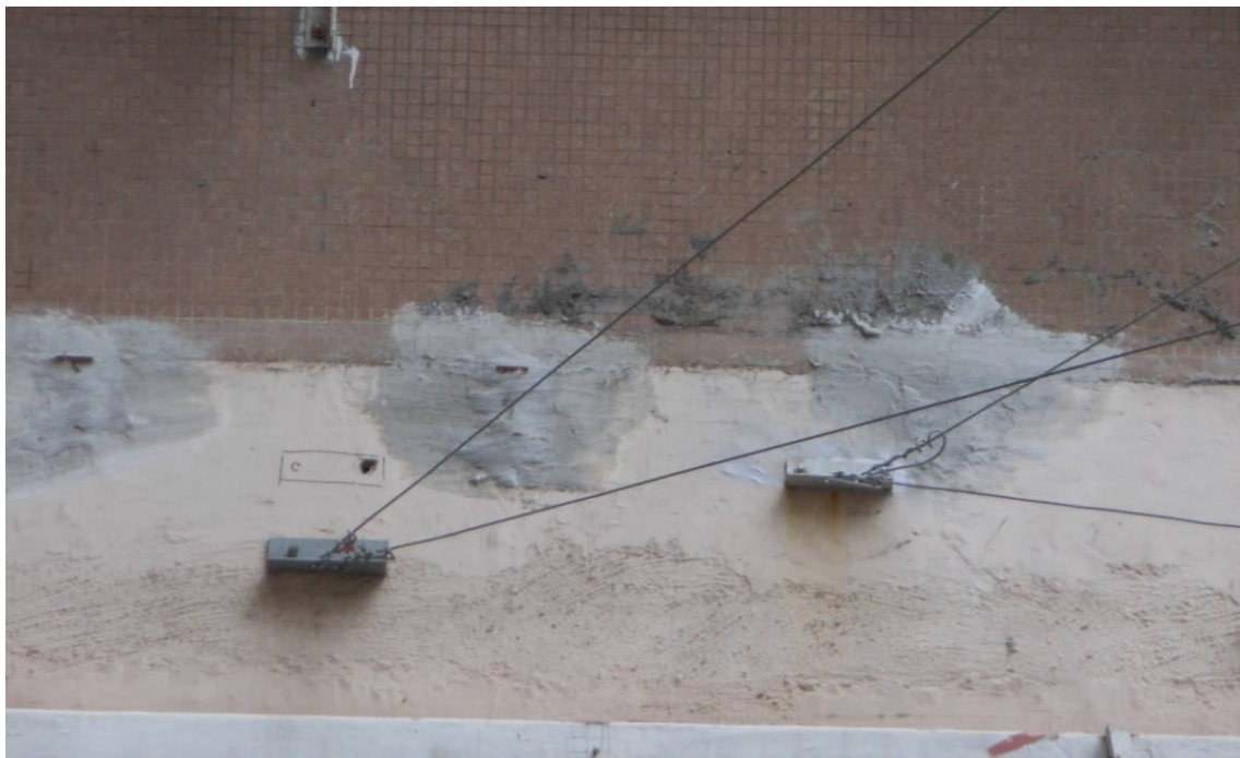
Photo 6: Anchor points B4 & B5 at the LHS of signboard
