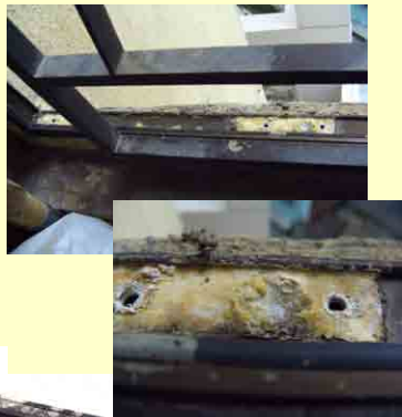
Greyish white powder at hinge
