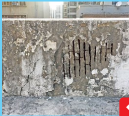
Cracks/exposed reinforcement
