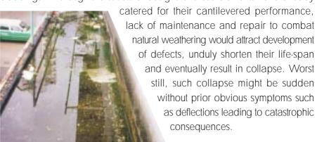
There are two main reasons why cantilevered structures demand close monitoring. Firstly, they are often exposed to weather attack or weakened by unauthorized building works. Secondly, unlike the conventional reinforced
