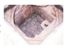
Foul air leaking from manholes could be stopped by repairing the edges of the manhole opening, cracks in the manhole and manhole cover or using a double-sealed type manhole cover.
