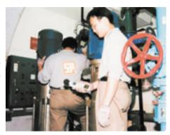
When the building management observes abnormal or excessive noise from ventilating or pumping systems, it should immediately identify the source and the cause for appropriate remedial measures.
