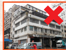
Subdivided units in industrial buildings are not suitable for domestic use
