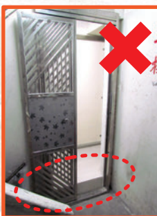
Thickening of the floor slab by laying solid screeding
