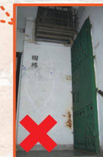
Opening formed in the staircase enclosure wall
