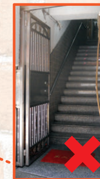
Metal gate obstructing the means of escape
