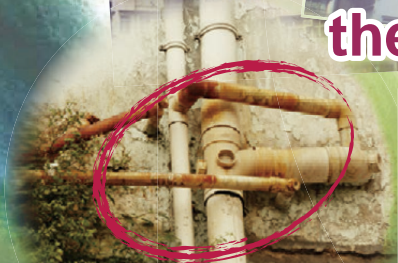
Check and repair drainage systems
