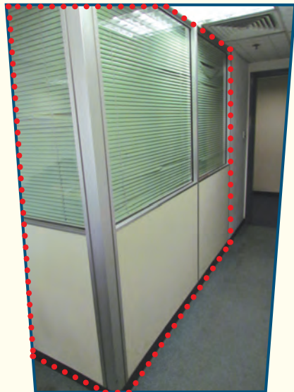
Lightweight partition board wall
