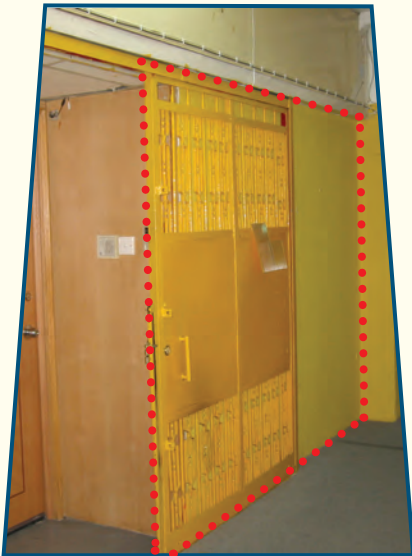
Metal gate of individual unit entrance not obstructing the means of escape
