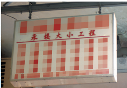
Signboard on or hung underneath the soffit of a balcony or canopy (other than a cantilevered slab)
