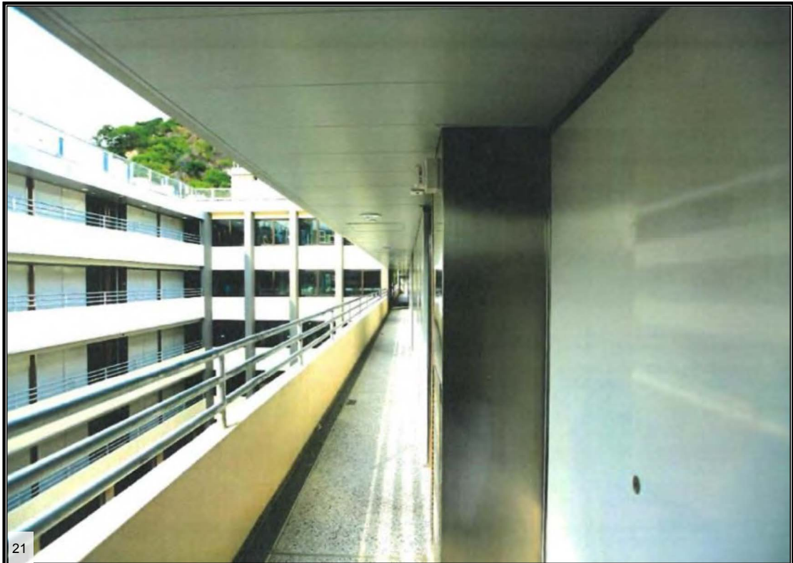
Parapet is rebuilt along corridors (Source: AD+RG)
