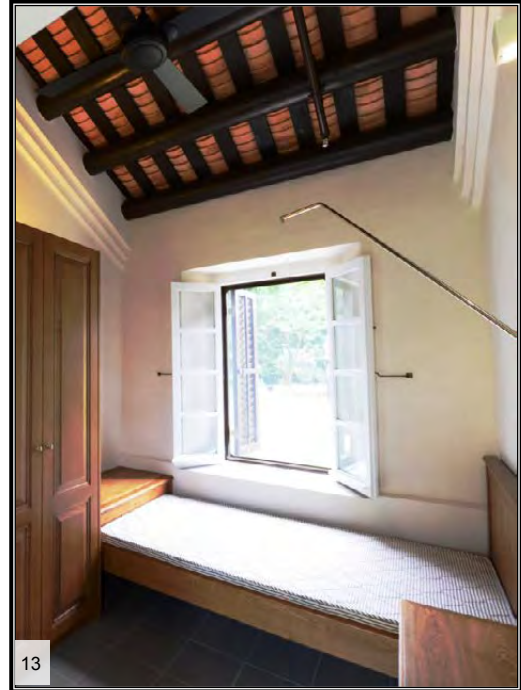
Reconstructed timber purlins and battens are protected with fire retardant paint
