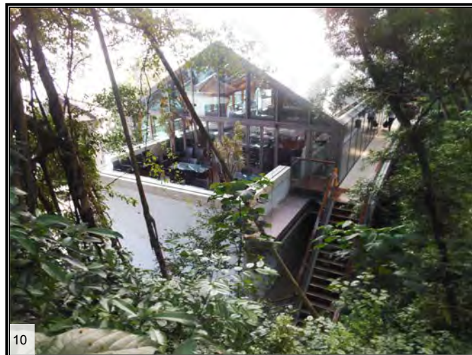
New staircase to the Annex
