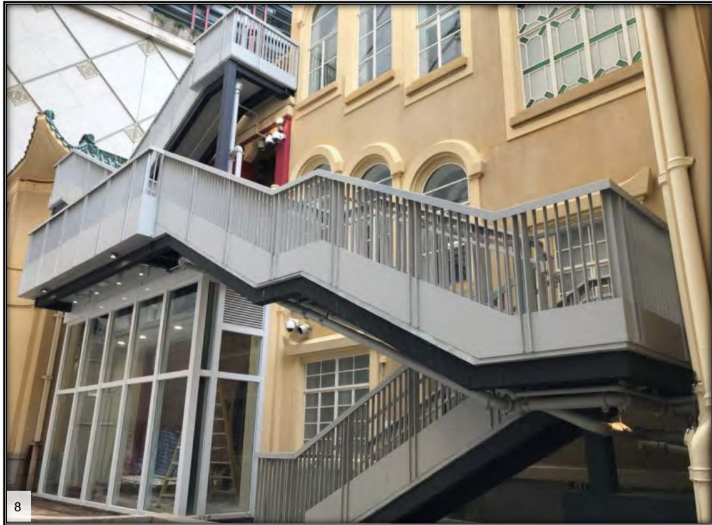
New open metal staircase (ST-4) added at the rear of HPM
