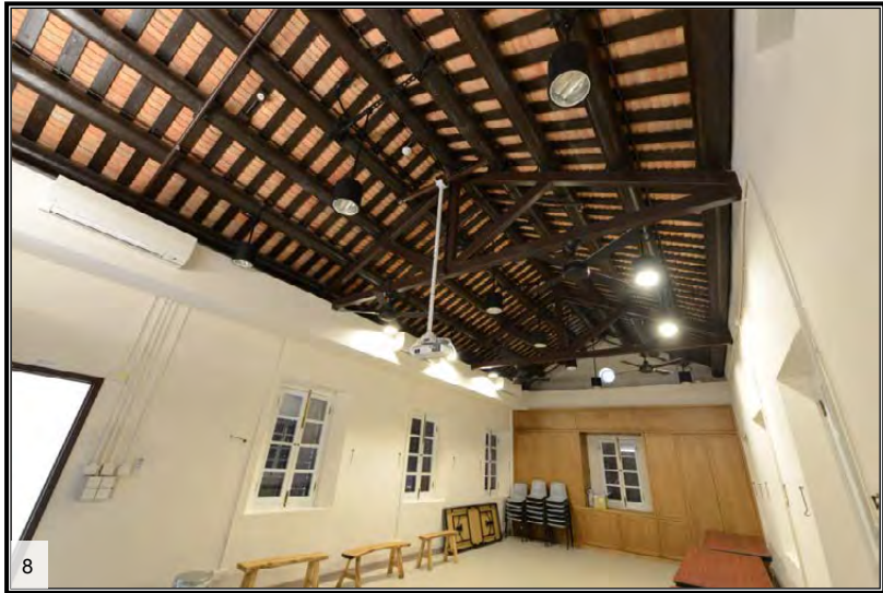
New timber roof for the multi-function room in the Main Building
