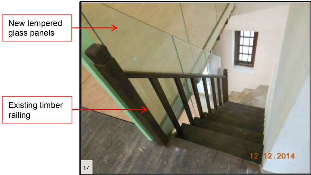
New protective barrier behind the existing sub-standard railing
