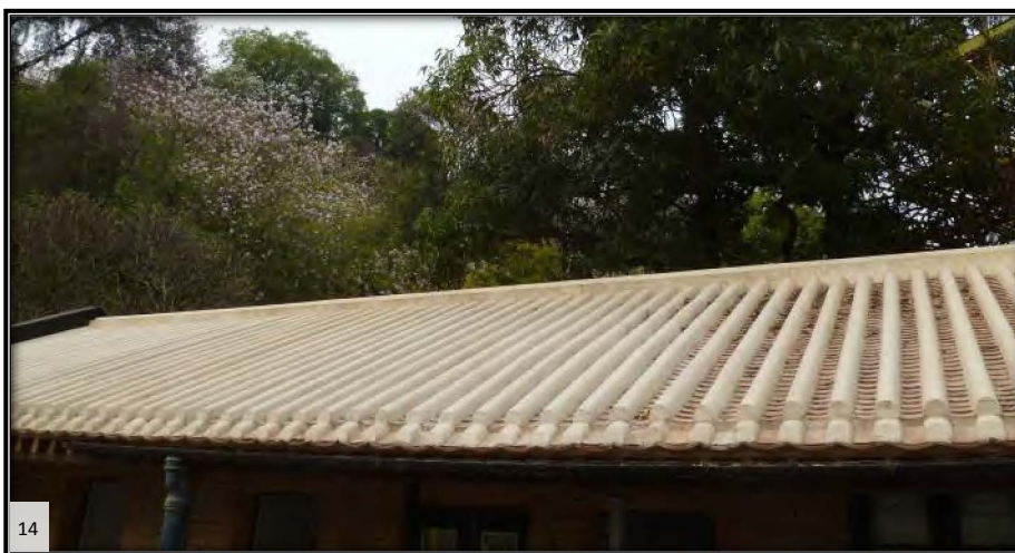
Timber pitched roof covered with non-combustible clay tiles
