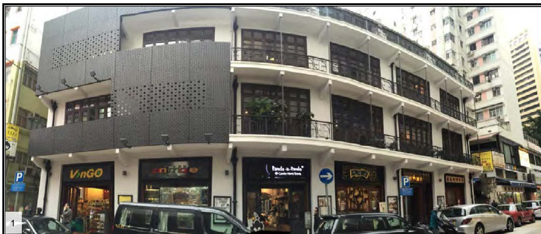
Elevation facing Mallory Street
