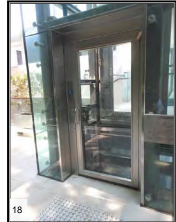
Vertical lifting platform to 1/F
