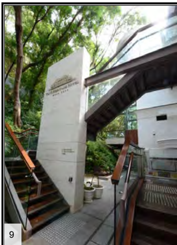
New staircase to the Main Building
