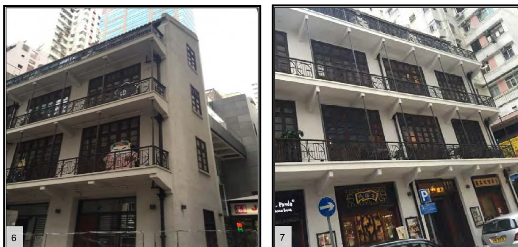
Reconstructed balconies facing Burrows Street and Mallory Street
