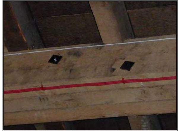
Photos 8 and 9 Three timber joists bolted together
