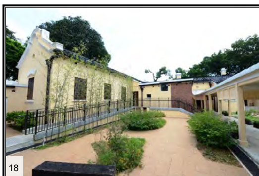
Ramp connecting the Main Building and courtyard
