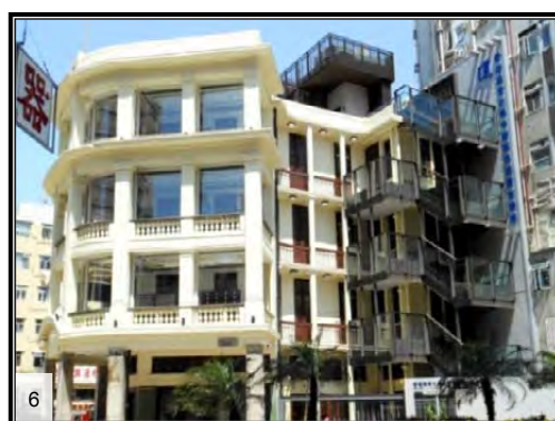
6 The new external staircase
