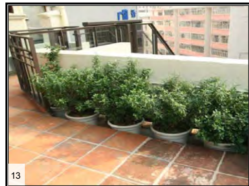
Potted plants to prevent users from getting close to low parapet walls
