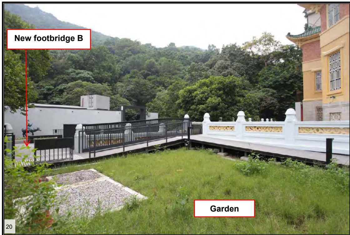
Photo of the Main Site (Source: Design 2 (HK) Limited)
