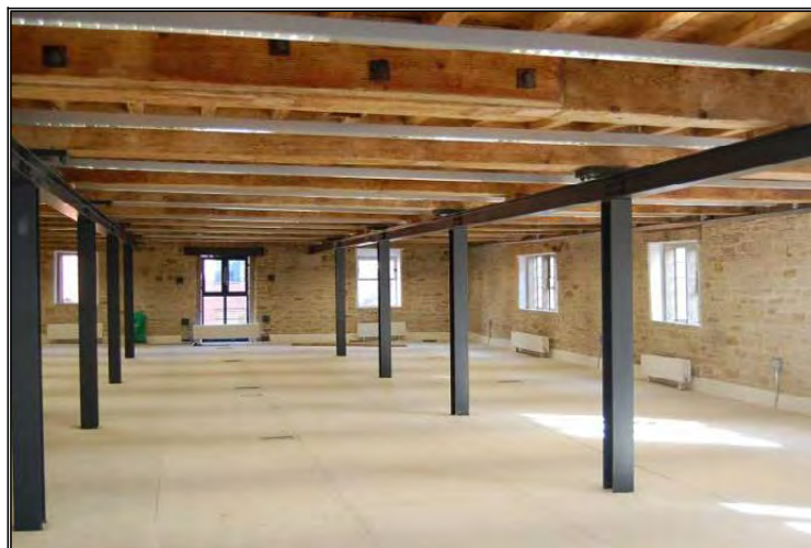
Photo 7 New beams and columns underneath the timber Joists
