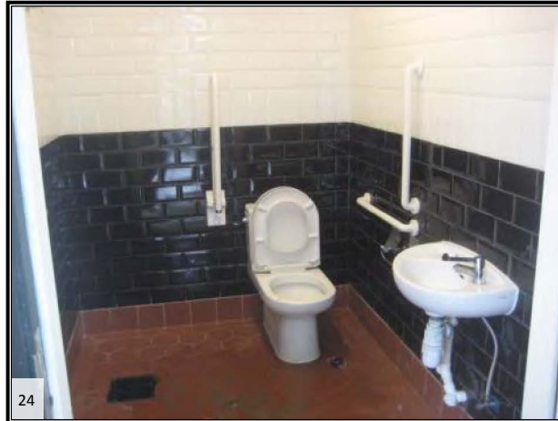
Other barrier free facilities, such as tactile guide path and accessible toilet
