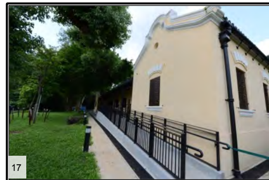
Ramp to the Main Building
