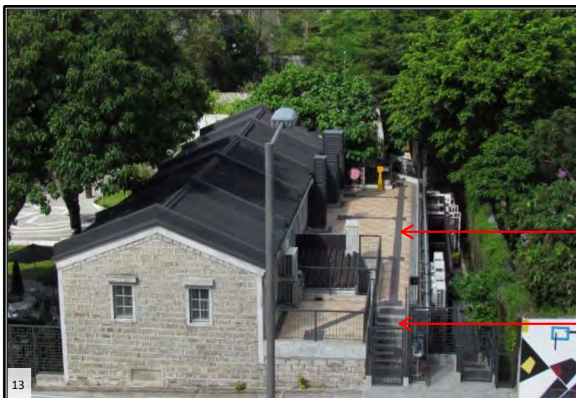
New metal deck connecting to open staircases
