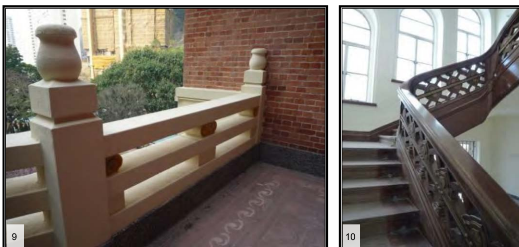
Existing parapets before revitalisation
