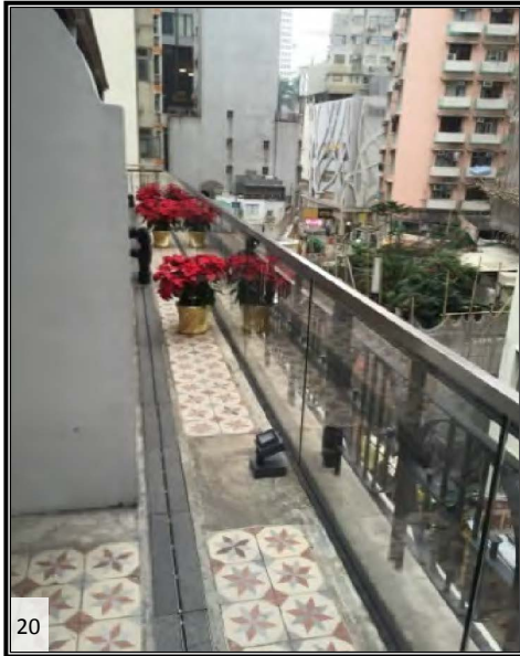
New glass balustrade added behind the existing railing at accessible balconies
