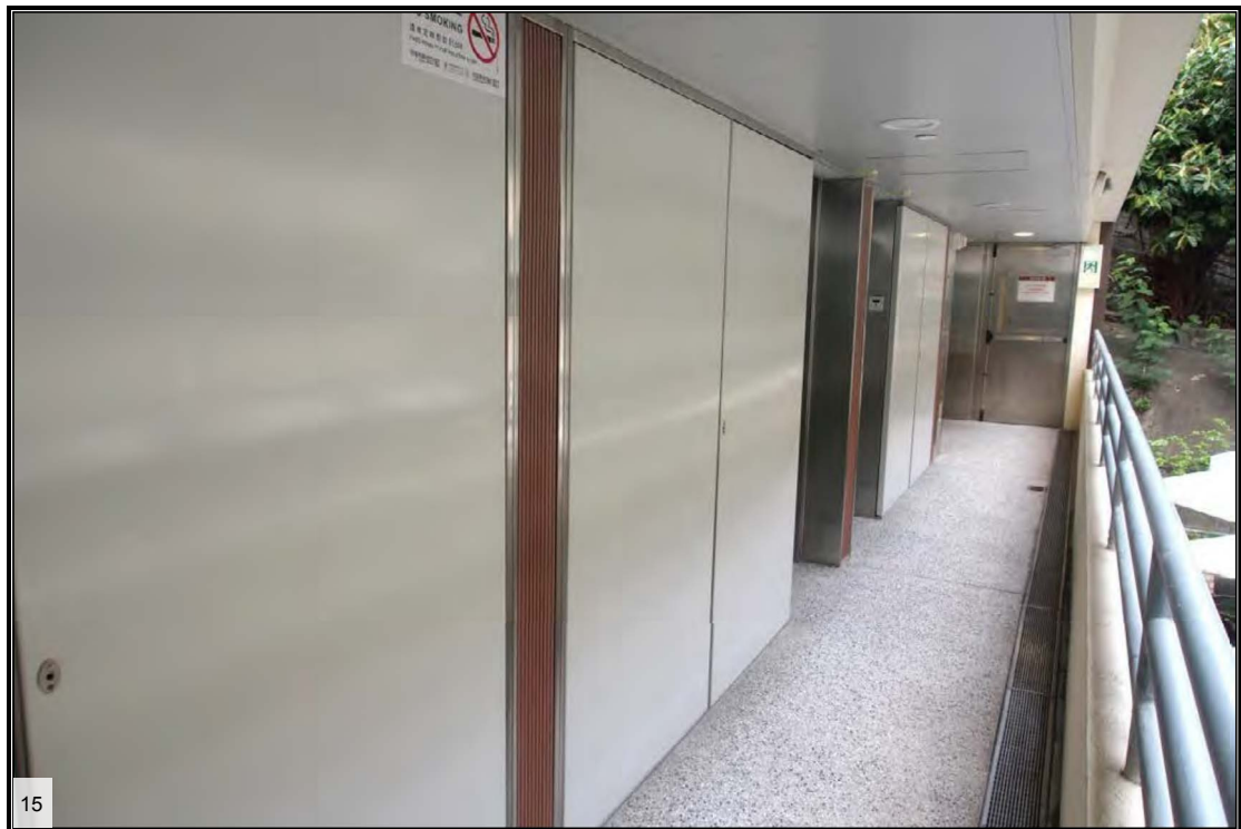
Access panels of pipe ducts facing the corridor
