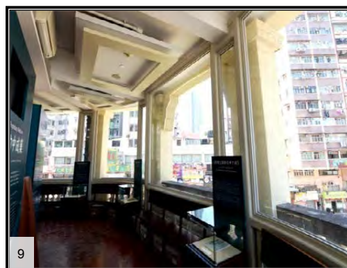
Enclosed verandah with new glass walls
