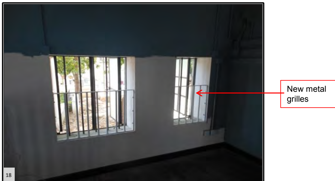
New metal grilles added at the existing window openings
