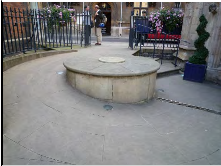
Photo 4 A circular access ramp to a church in Cambridge, UK
