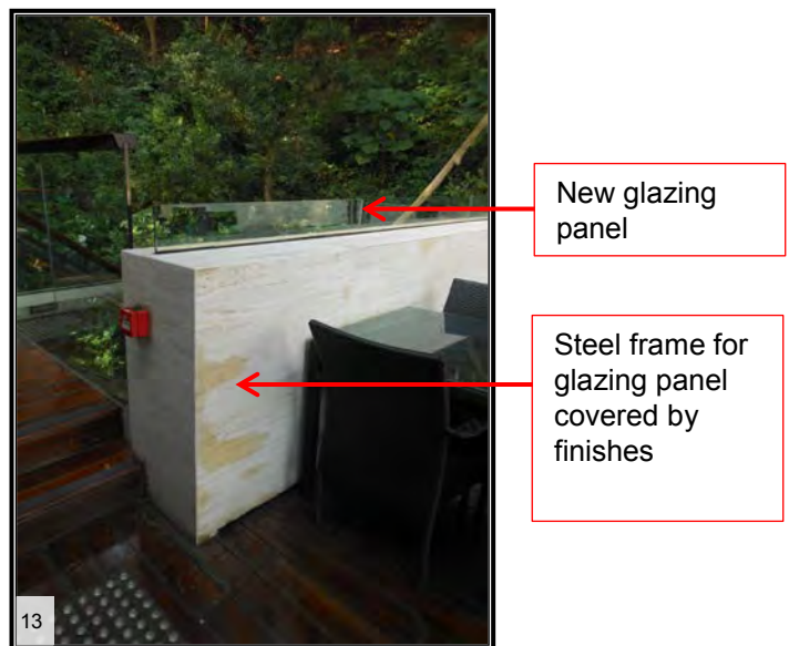
Additional glazing panel at Annex
