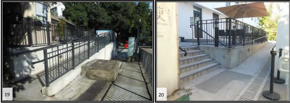
New Accessible ramps at the entrance and other locations within the site
