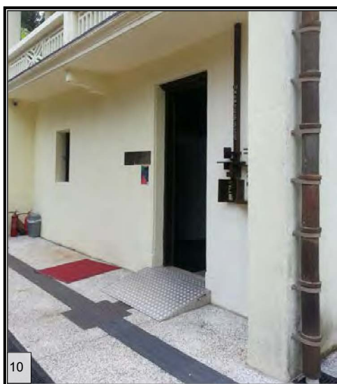
Tactile warning strips and movable ramp at G/F entrance
