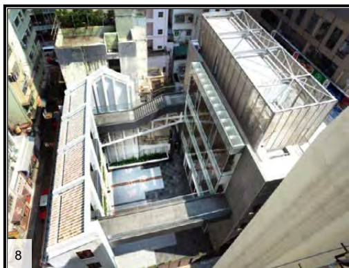
Aerial photo showing the trusses connecting the New Annex and the existing facade
