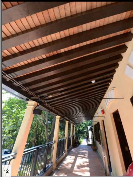
Existing timber purlins and battens are protected with fire retardant paint
