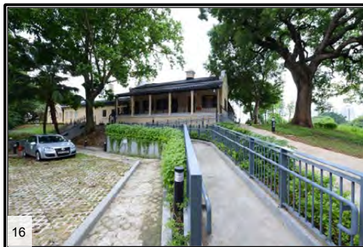
Initial access ramp to the compound
