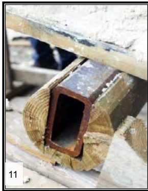
11 New steel members embedded in timber purlin
