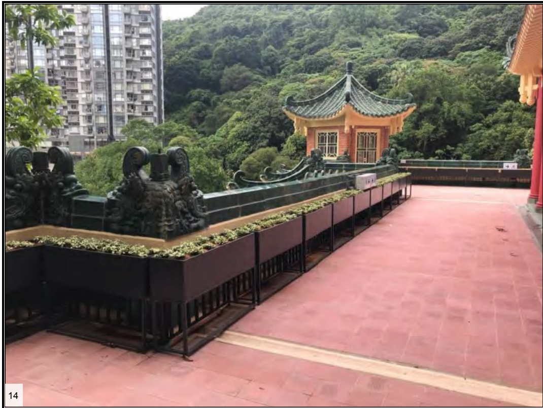
Type 2 pot planters along the parapet of the roof
