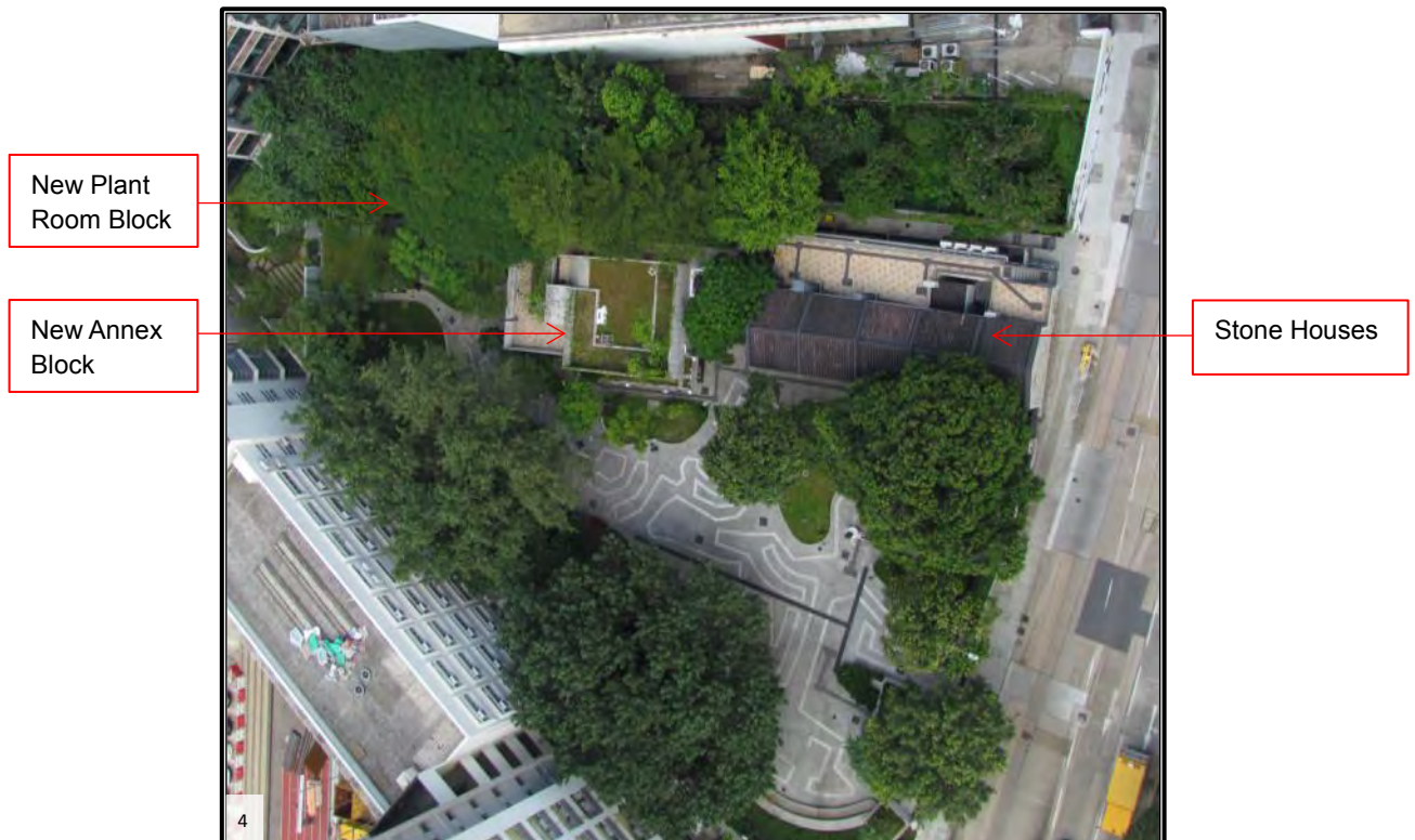
Stone Houses, New Annex Block and Plant Room
