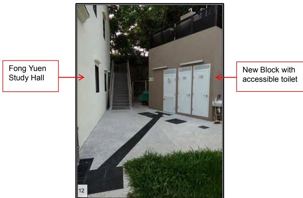
Provision of accessible toilet
