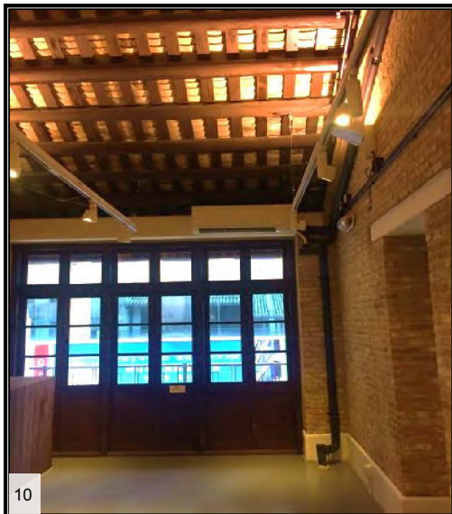
The Chinese-style tiled and timber roof
