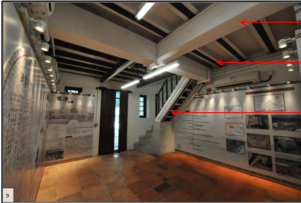
Timber staircase and timber floor of Interpretation Centre strengthened with steel beams and stringers
