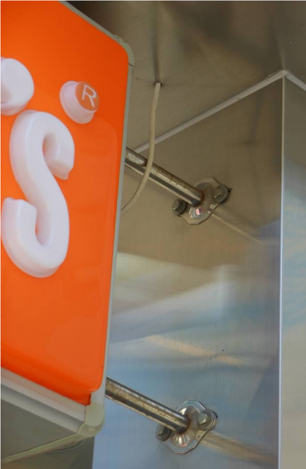
Photo 3: Fixing points of signboard
