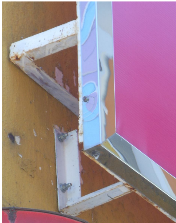
Photo 3: Fixing points A7 of signboard (fixing points A1, A4 & A10 are similar)
