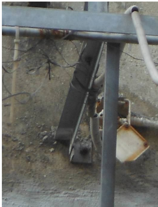
Photo 3: Fixing points B2 of signboard (fixing points A1-A6, B1, B3-B6 are similar)
