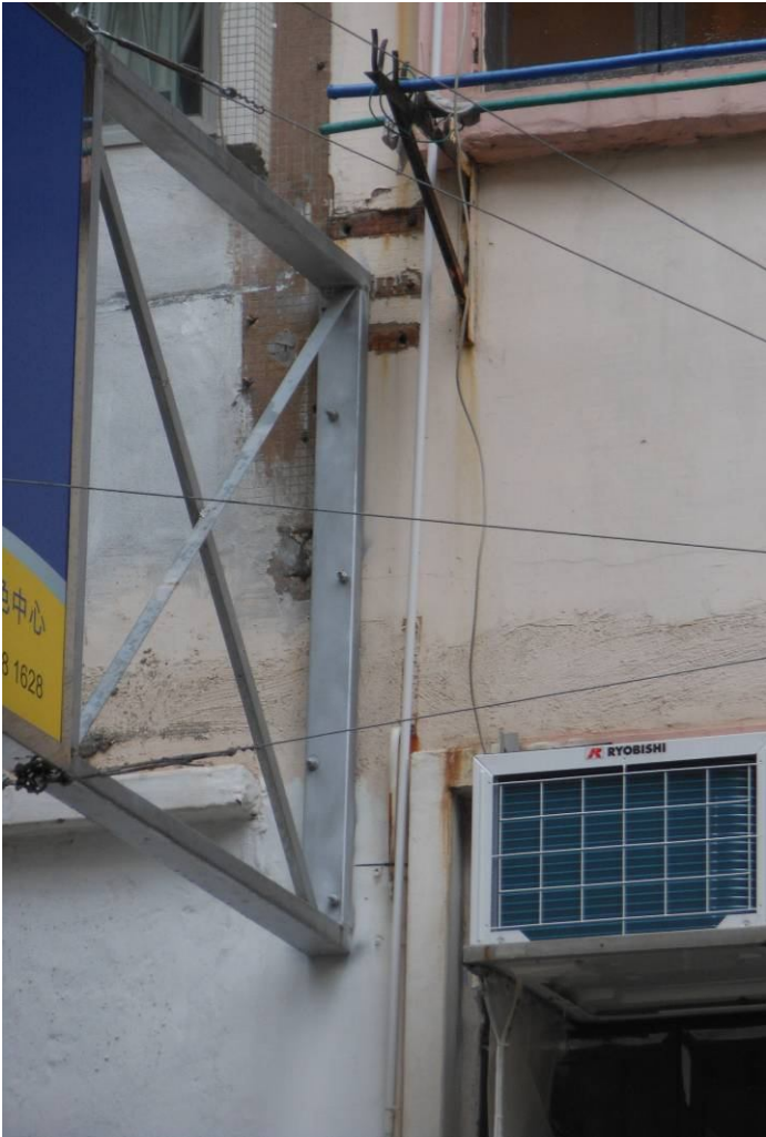
Photo 3: Fixing points A1-A5 of signboard
