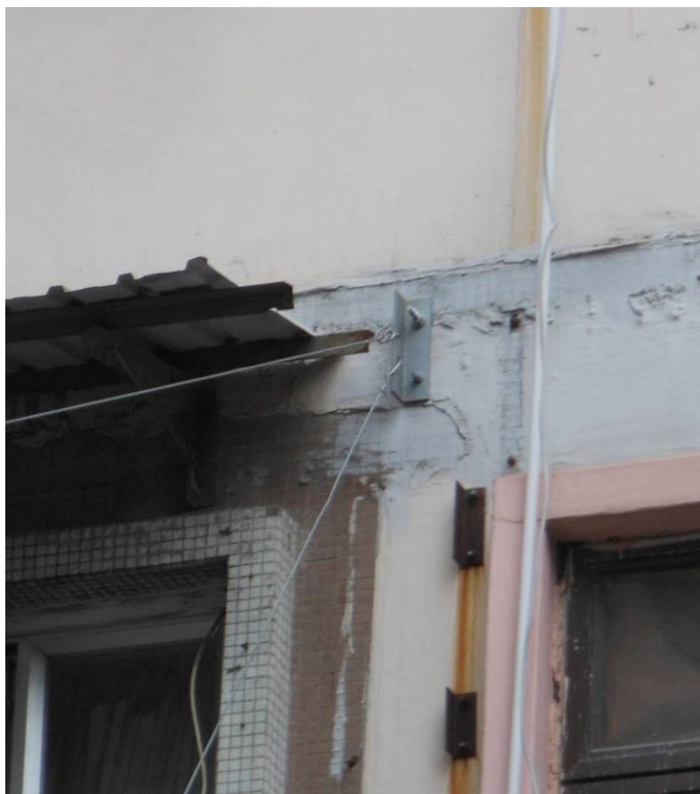
Photo 4: Anchor point B1 at the top of signboard
