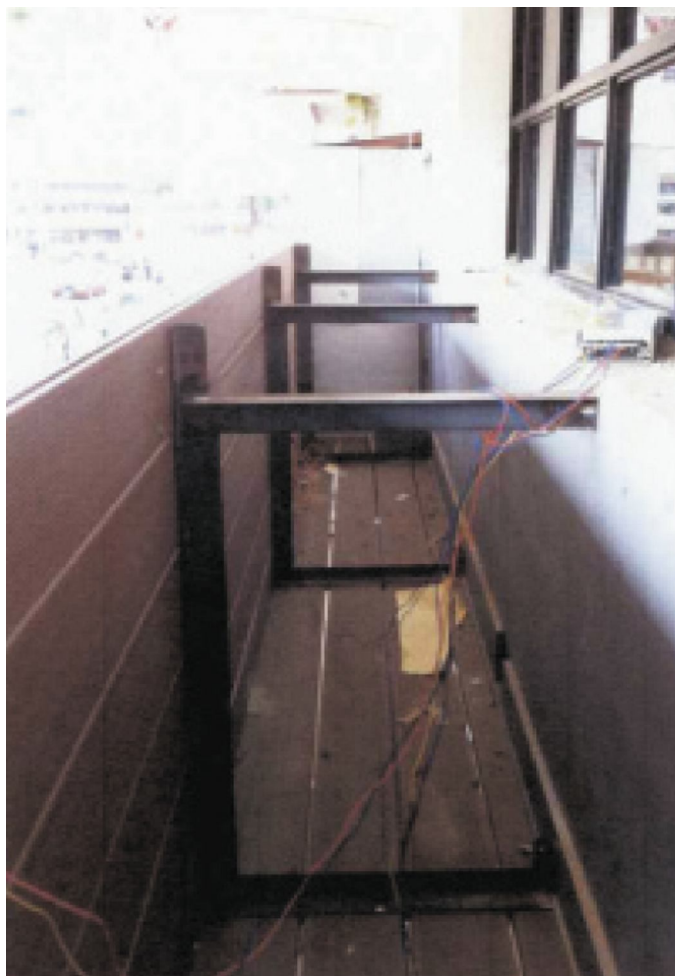
Photo 3: Fixing points of signboard (other fixing points are similar)
