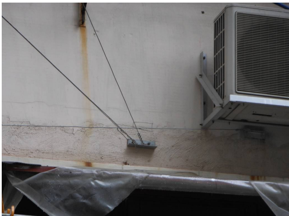
Photo 5: Anchor points B2 & B3 at the RHS of signboard
