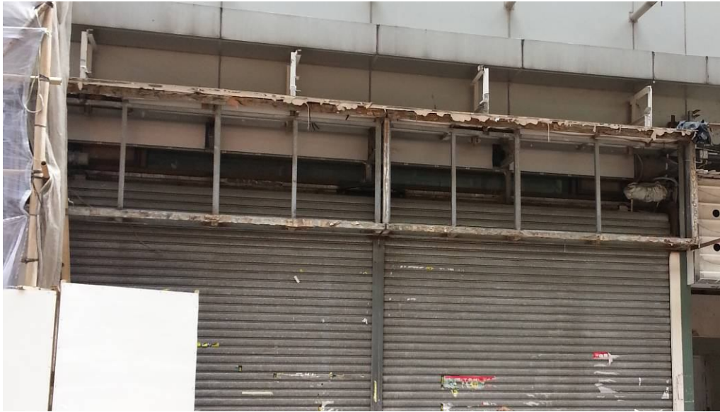
Photo 3: Fixing points B2 of signboard (fixing points A1-A6, B1, B3-B6 are similar)
