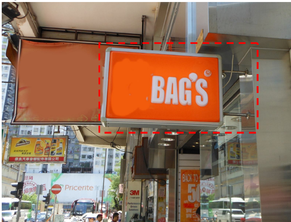
Photo 1: Signboard front view
