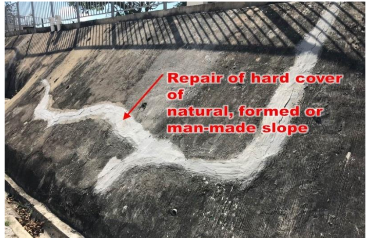
Item 3.53 Repair of hard cover of natural, formed or man-made slope
