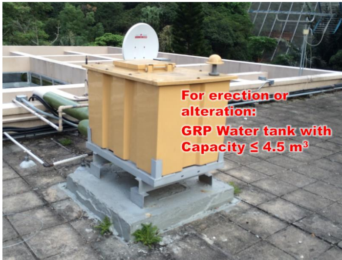
Item 1.49 Erection or alteration of GRP water tank
