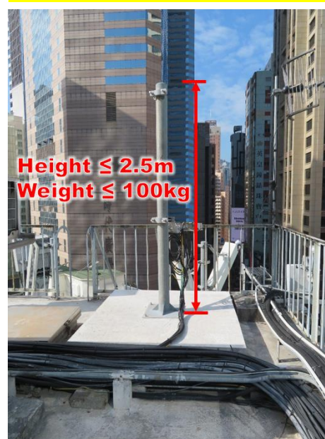
Item 2.54 Erection or alteration of pole on roof
