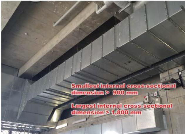
Item 1.46 Erection or alteration of metal ventilation duct inside building
