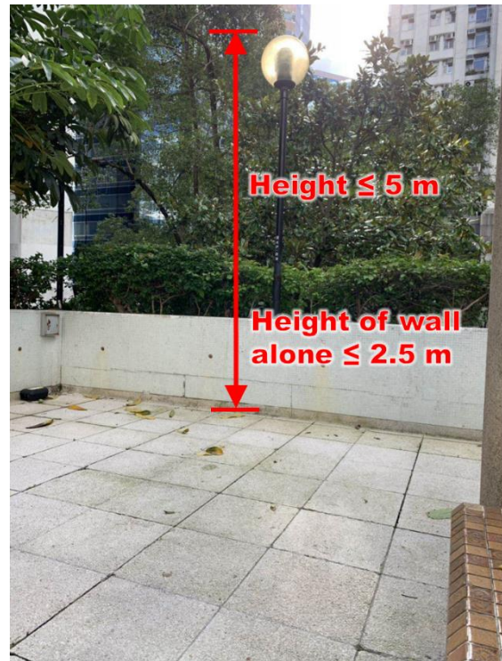
Item 2.57 Erection of pole on top of a solid fence wall on-grade
