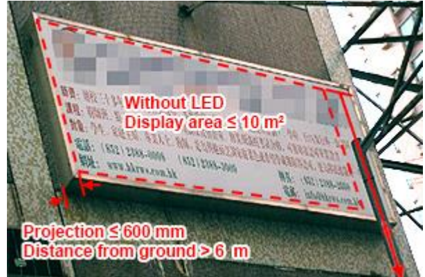
Item 2.19 Erection or alteration of wall signboard
