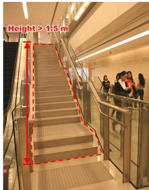
Item 1.32 Removal of internal staircase
