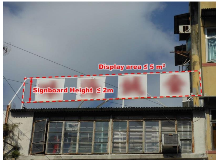
Item 3.19 Removal of signboard on roof
