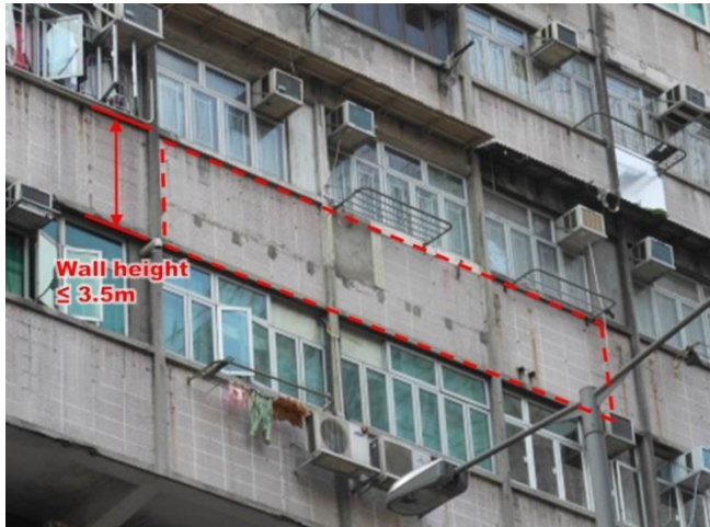
Item 3.12 Repair of non-load bearing block wall
