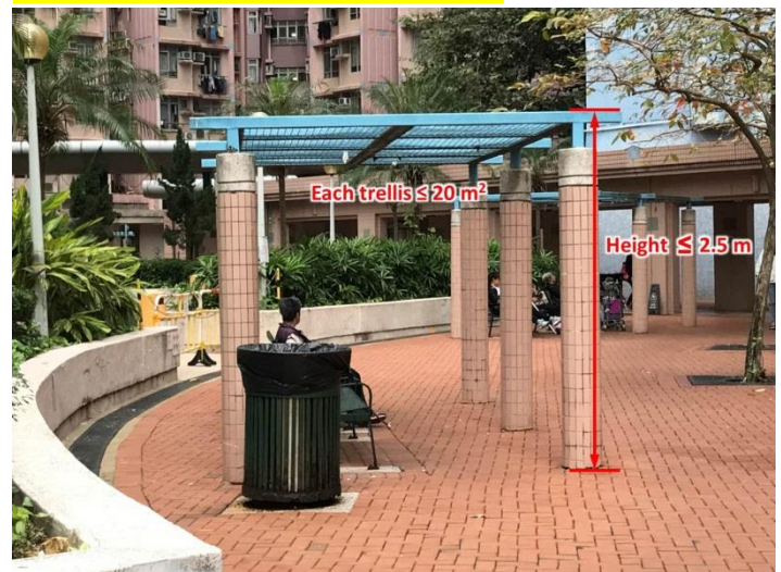
Item 3.44 Repair of trellis on grade
