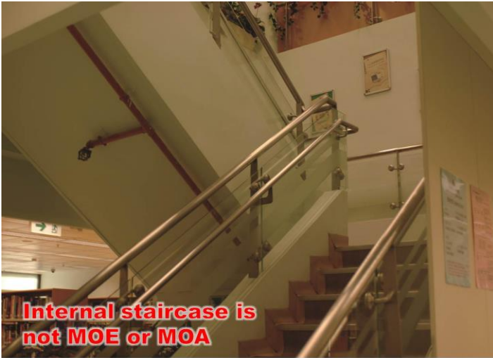
Item 1.1 Erection or alteration of internal staircase
