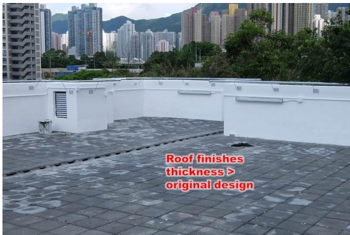
Item 1.62 Laying and repair of roof finished
