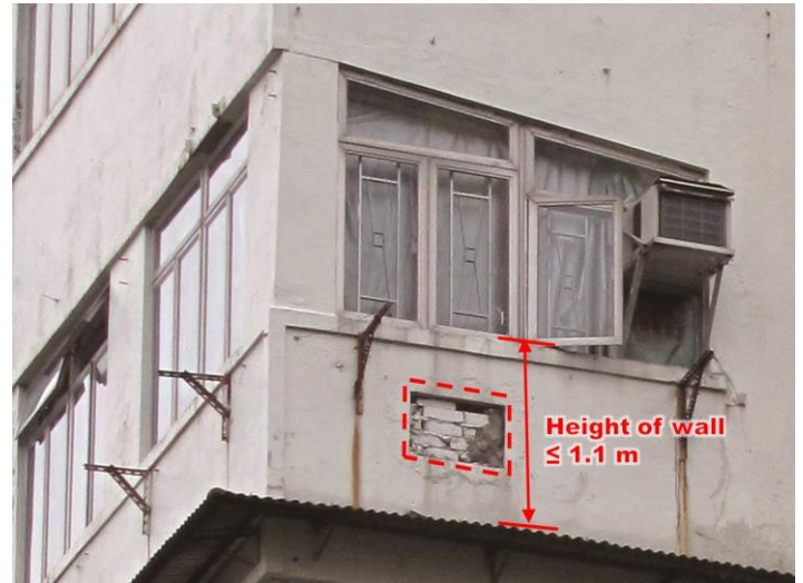
Item 3.11 Erection, alteration or removal of non-load bearing block wall
