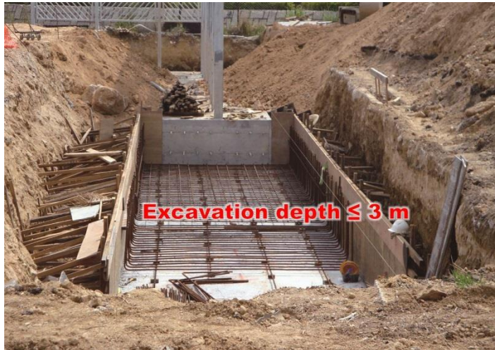
Item 1.11 Construction or alteration of spread footing
