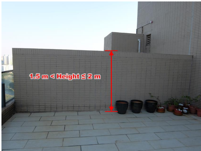
Item 2.64 Removal of solid fence wall on roof
