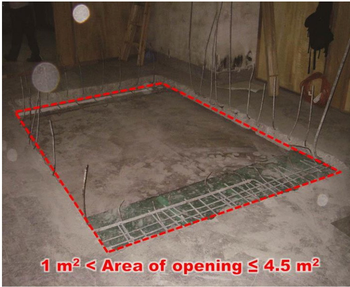
Item 1.35 Reinstatement of slab
