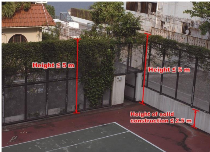
Item 3.5 Removal of external mesh fence on-grade
