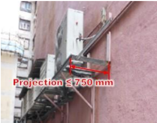
Item 1.28 Erection, alteration or removal of supporting frame for BSI
