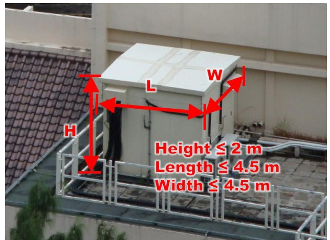
Item 3.8 Removal of radio base station
