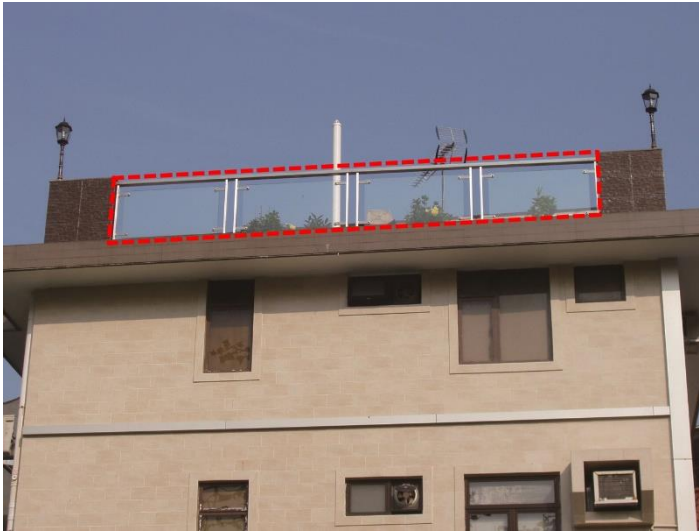
Item 1.6 Erection, alteration or removal of protective barrier
