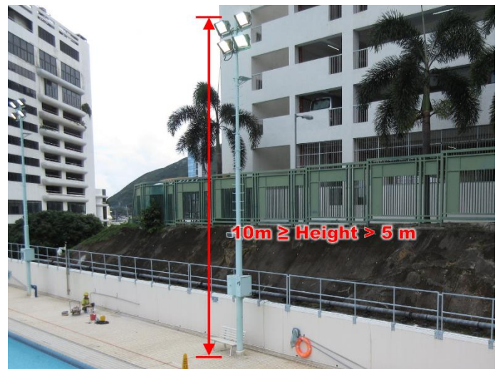
Item 2.66 Removal of external pole on-grade
