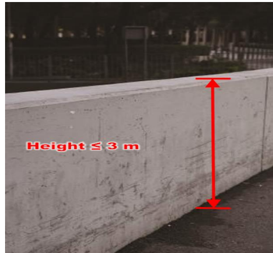
Item 2.6 Erection or alteration of fence wall on-grade
