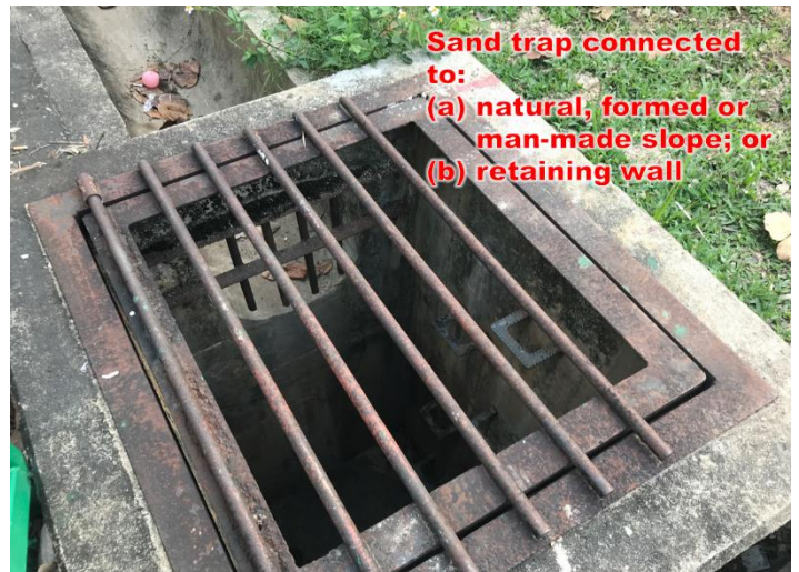
Item 3.53 Repair of sand trap
