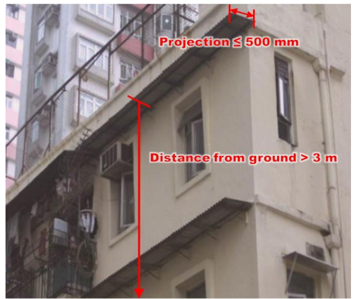
Item 3.25 Erection or alteration of canopy
