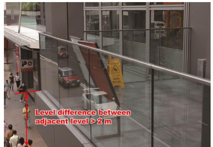
Item 2.5 Repair or replacement of protective barrier
