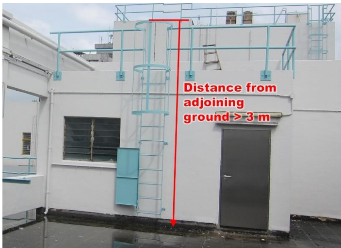
Item 3.51 Repair or Removal of external cat ladder
