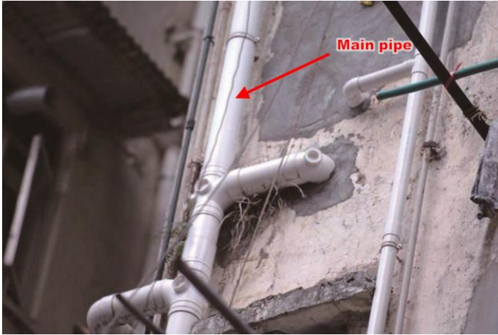
Item 2.30 Erection, repair, alteration or removal of aboveground drainage
