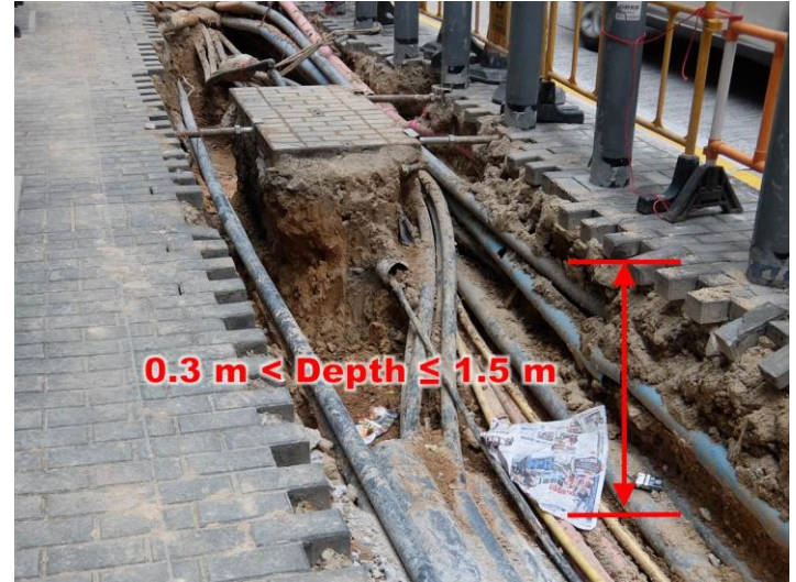
Item 2.11 Excavation works
