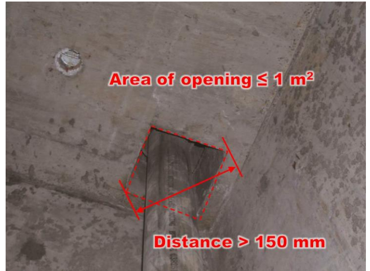
Item 2.35 Reinstatement of slab
