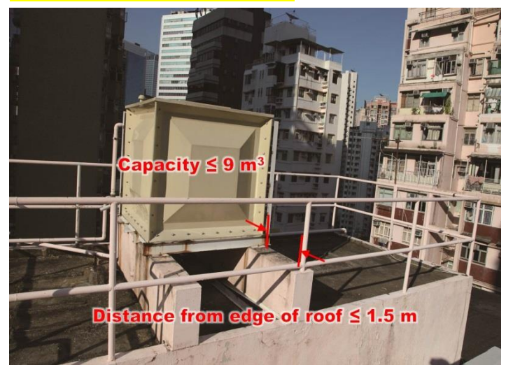
Item 2.4 Removal of water tank
