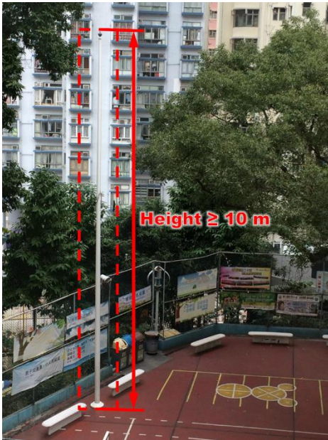
Item 1.10 Removal of external pole on-grade
