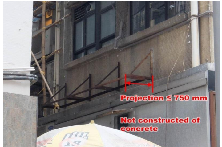
Item 3.26 Removal of rack
