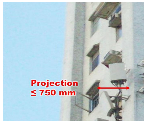
Item 1.28 Erection, alteration or removal of supporting frame for BSI
