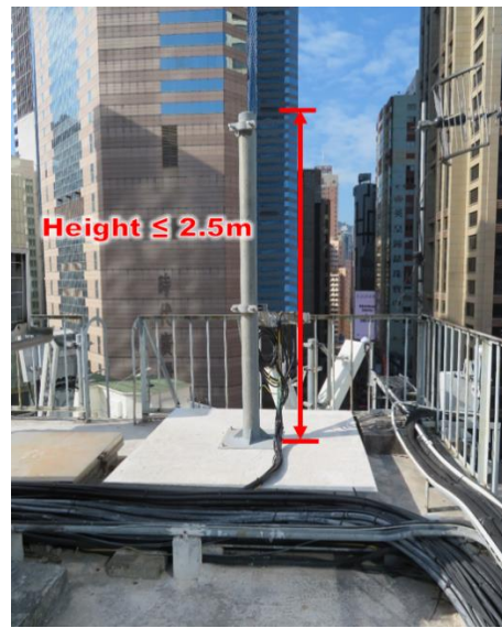
Item 3.60 Repair of pole on roof.
