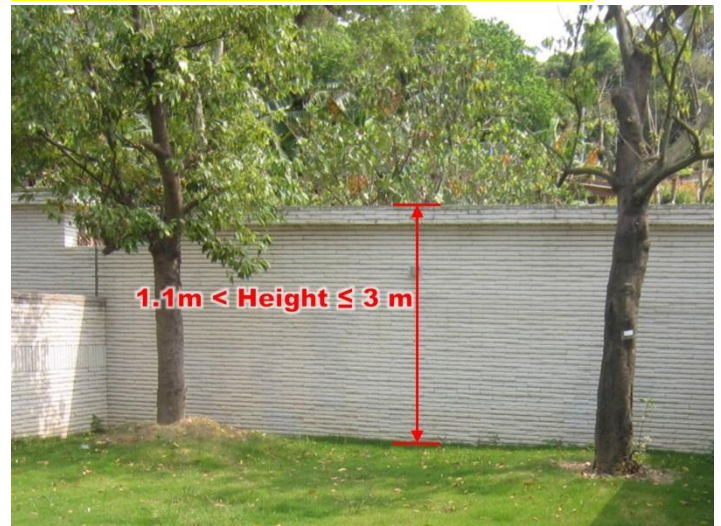
Item 3.57 Repair of solid fence wall on-grade
