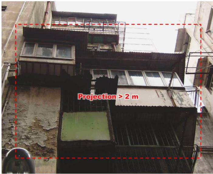
Item 1.30 Removal of unauthorised structure
