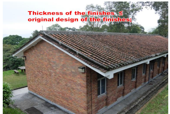
Item 2.34 Laying, repair or removal of roof finishes
