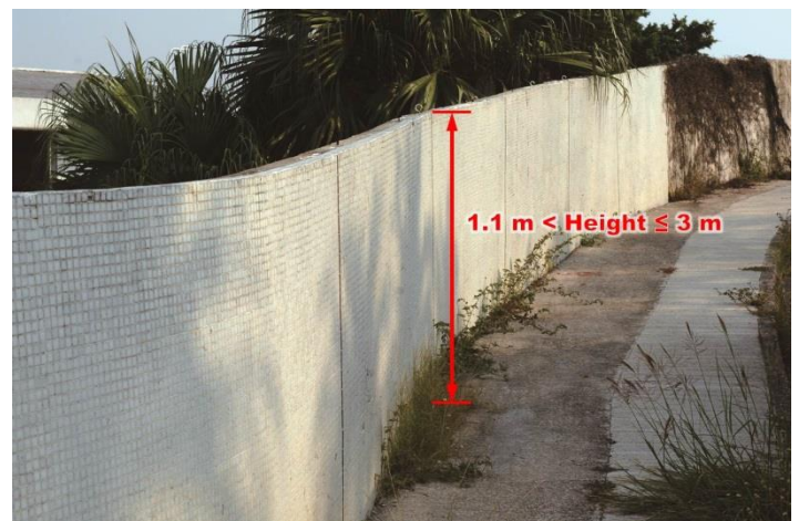
Item 3.4 Removal of solid fence wall on-grade
