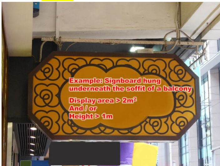
Item 2.27 Removal of signboard hung underneath balcony
