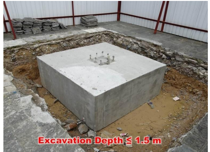
Item 2.10 Construction or alteration of spread footing
