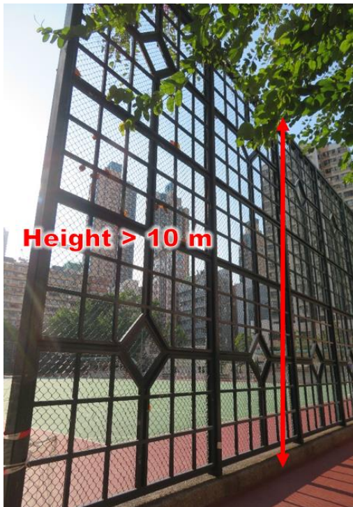
Item 1.10 Removal of external mesh fence on-grade
