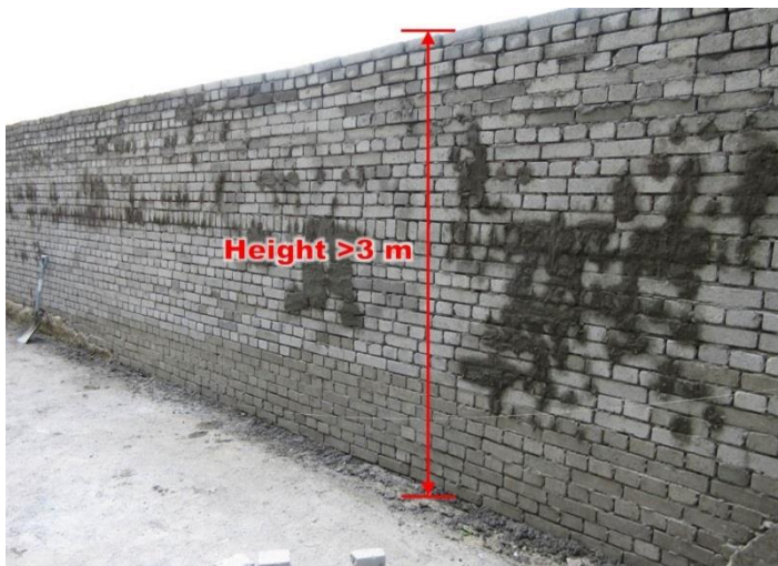
Item 1.57 Repair of solid fence wall on-grade
