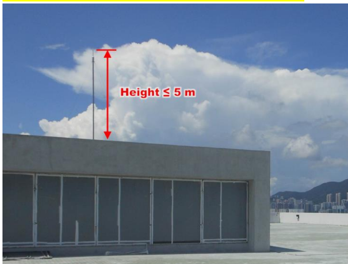
Item 1.54 Erection or alteration of pole on roof
