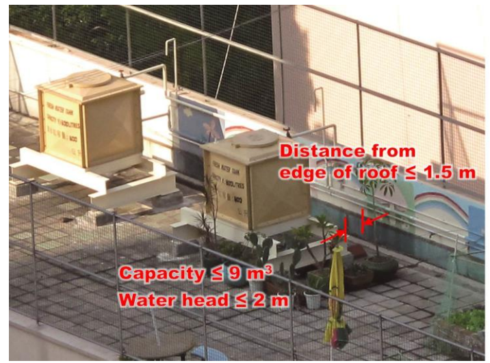
Item 2.3 Replacement of GRP water tank
