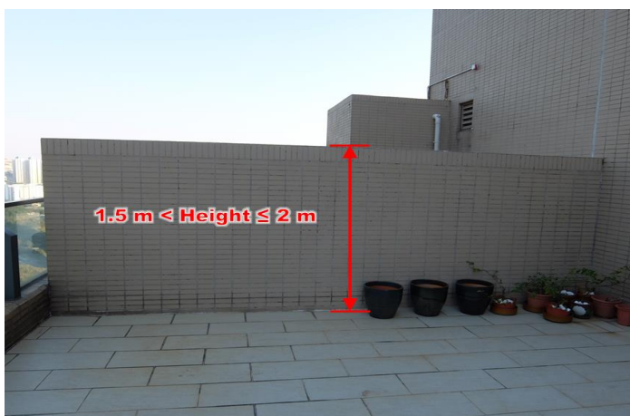
Item 2.61 Repair of solid fence wall on roof
