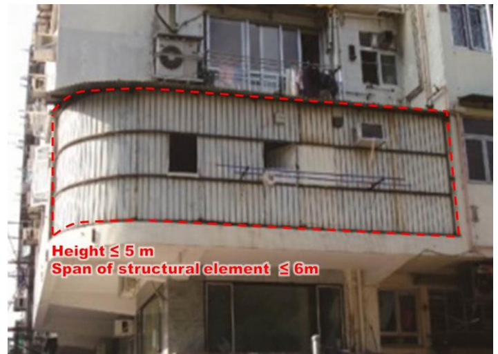
Item 2.39 Removal of unauthorised structure
