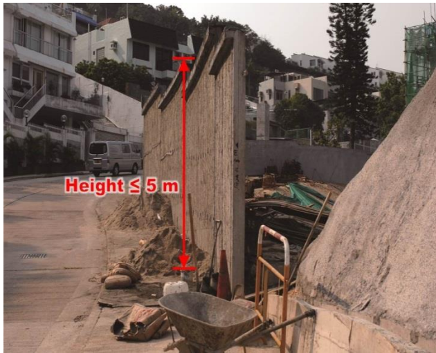
Item 1.7 Erection or alteration of fence wall on-grade
