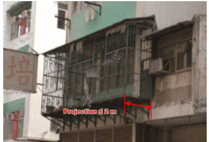
Item 2.32 Removal of unauthorised structure
