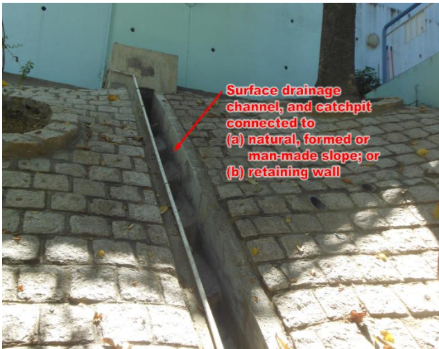
Item 3.53 Repair of surface drainage channel or catchpit
