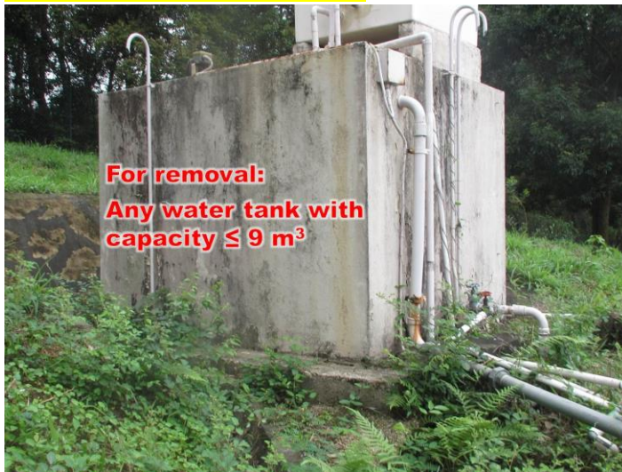
Item 2.4 Removal of water tank
