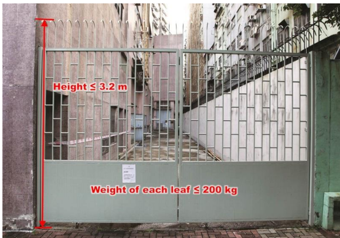
Item 3.33 Removal of metal gate
