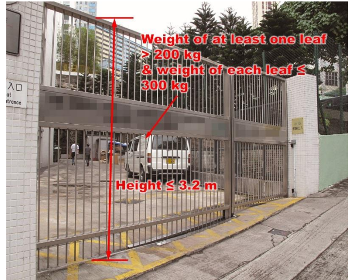
Item 2.16 Erection, alteration or repair of metal gate
