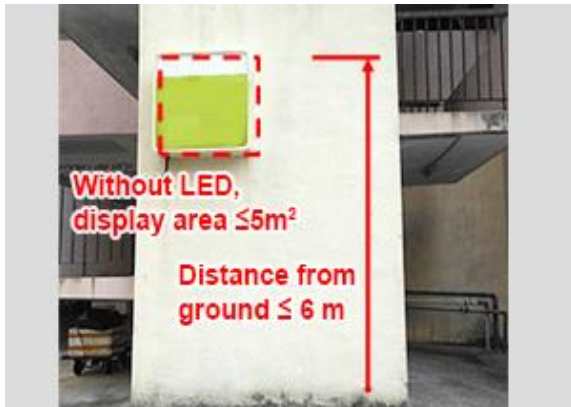
Item 3.17 Erection, alteration or removal of wall signboard
