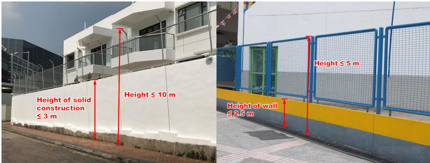
Item 2.7 Erection or alteration of mesh fence on-grade
