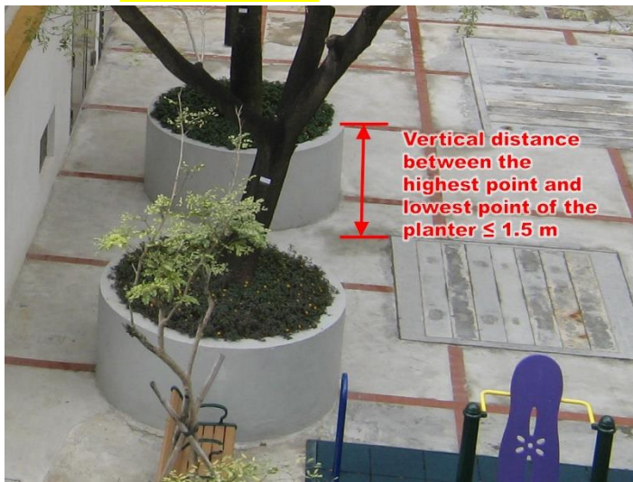
Item 2.52 Erection, alteration, repair or removal of planter on-grade
