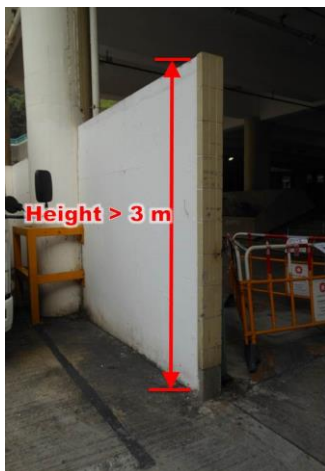
Item 1.9 Removal of solid fence wall on-grade
