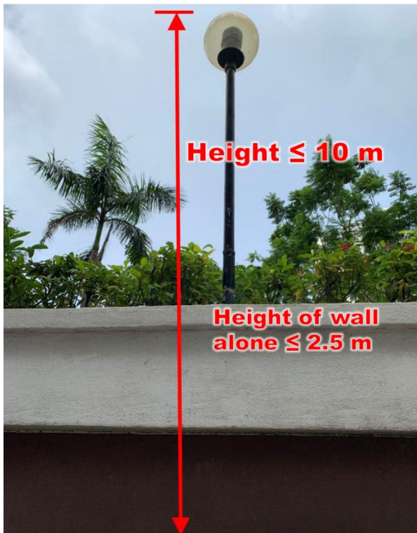
Item 1.59 Erection of pole on top of a solid fence wall on-grade
