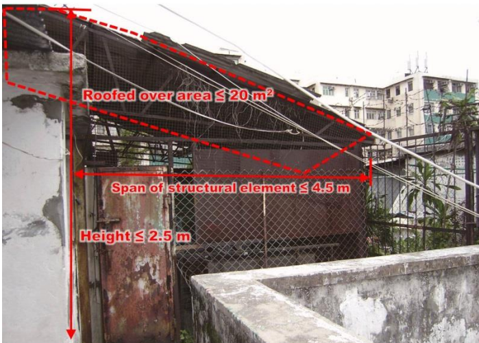
Item 3.32 Removal of unauthorised structure
