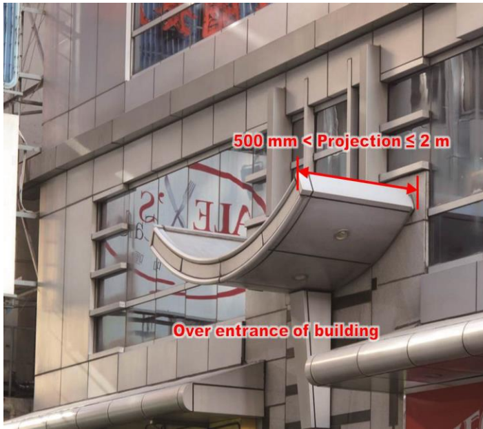
Item 1.27 Erection, alteration or removal of canopy
