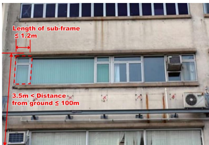
Item 3.6 Construction, alteration, repair or replacement of window or window wall
