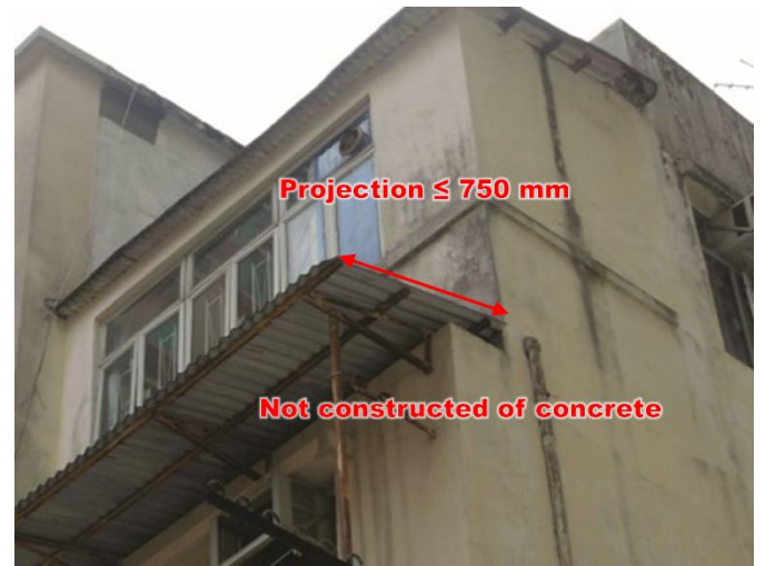
Item 3.26 Removal of canopy
