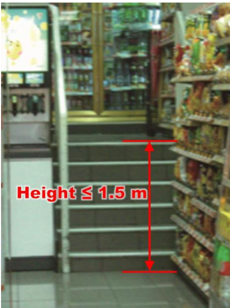
Item 3.1 Removal of internal staircase
