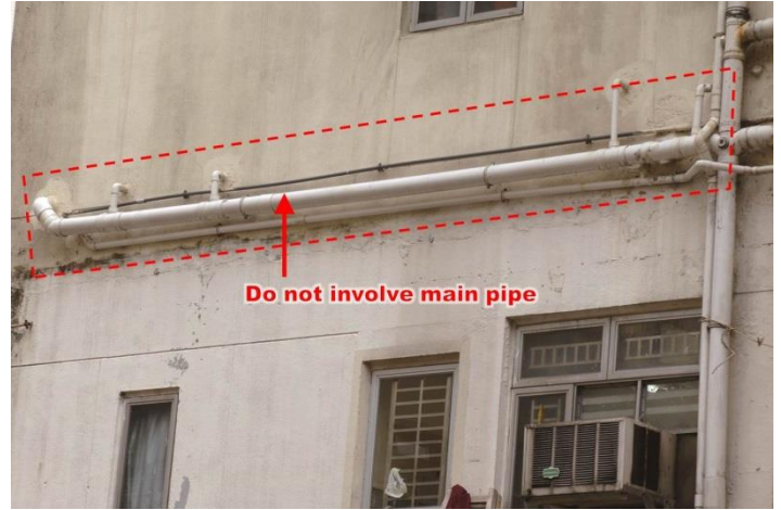
Item 3.23 Erection, repair, alteration or removal of aboveground drainage
