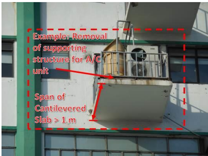
Item 1.5 Removal of supporting structure or metal casing for BSI
