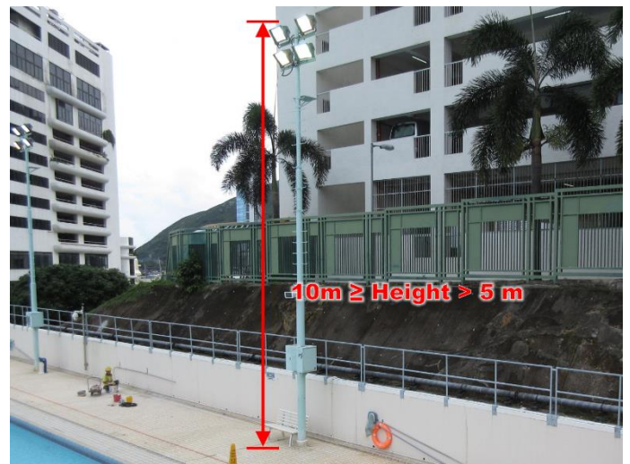
Item 2.59 Repair of external pole on-grade
