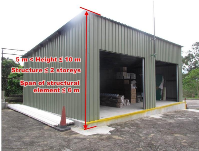
Item 1.38 Removal of unauthorised structure
