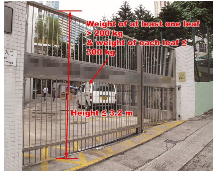
Item 2.40 Removal of metal gate
