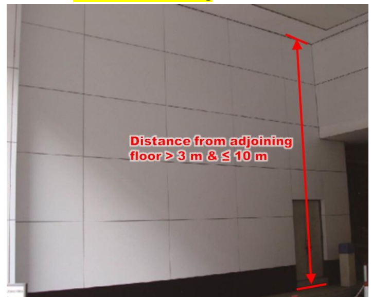
Item 2.33 Erection, Repair or removal of panel on a wall inside a building
