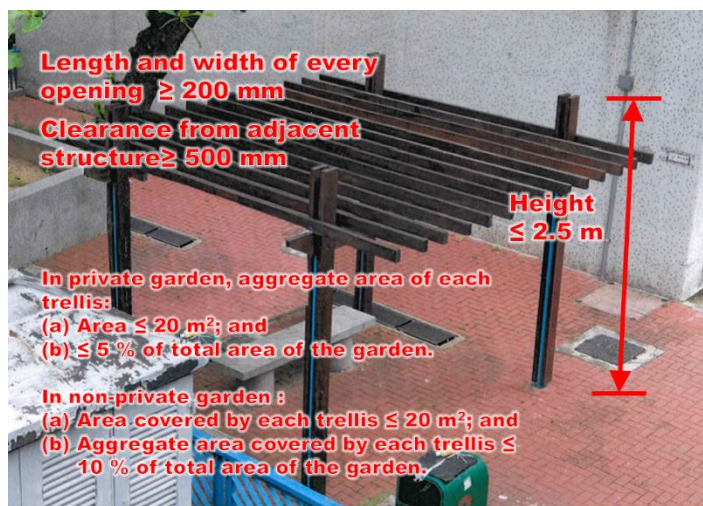
Item 2.44 Erection or alteration of trellis on grade
