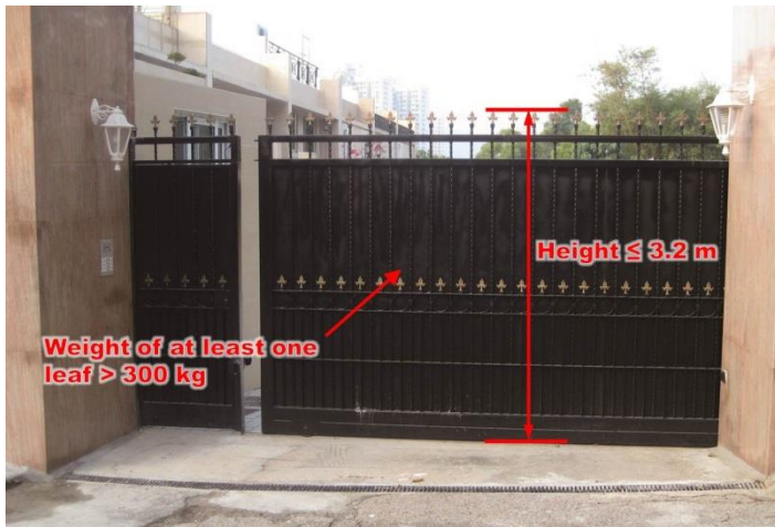
Item 1.40 Removal of metal gate
