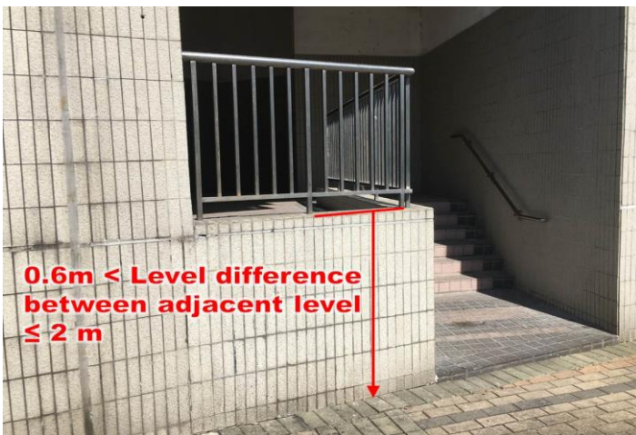
Item 3.3 Repair or replacement of protective barrier
