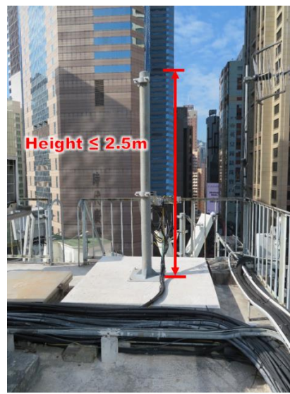
Item 3.63 Removal of pole on roof
