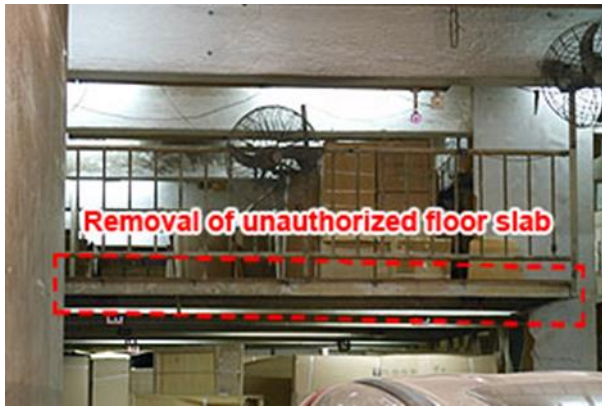
Item 1.39 Removal of unauthorised floor slab
