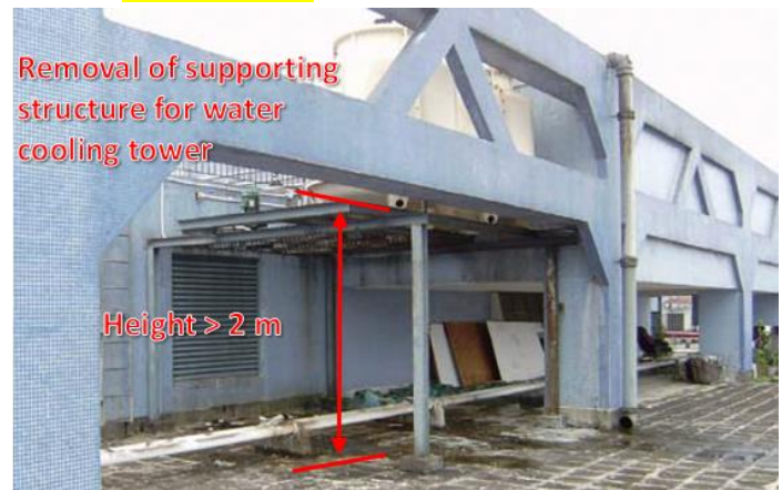
Item 2.2 Removal of supporting structure or metal casing for BSI
