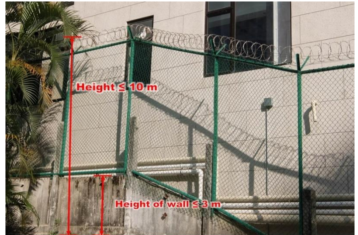
Item 2.67 Removal of external mesh fence on-grade
